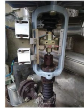
Picture: Meerhout Actuator Assembly
